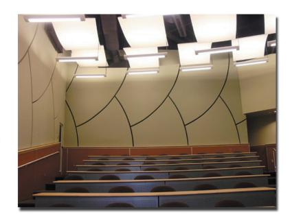
Ceiling clouds are available in 1/2", 1", 1 1/2" or 2" thickness with maximum sizes up to 4'x 10'.
