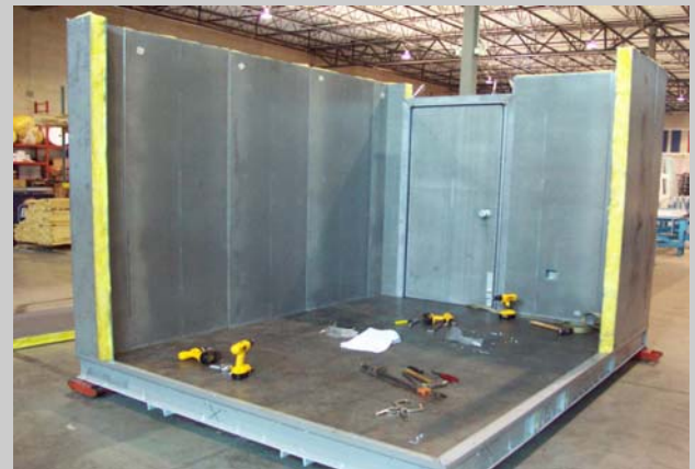
Modular Wall Panels Being Assembled Onto Base
