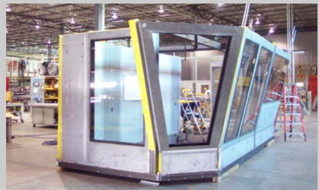
Custom Cantilevered Walls & Windows Being Assembled
