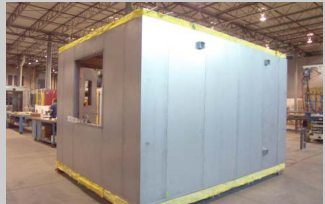
Assembled Structure Ready for Finishing Trim
